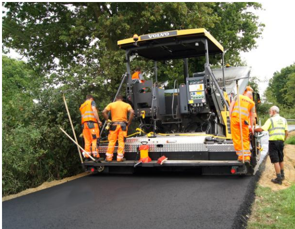
Asphalt paving of Potsdamer Weg with the new Volvo paver
